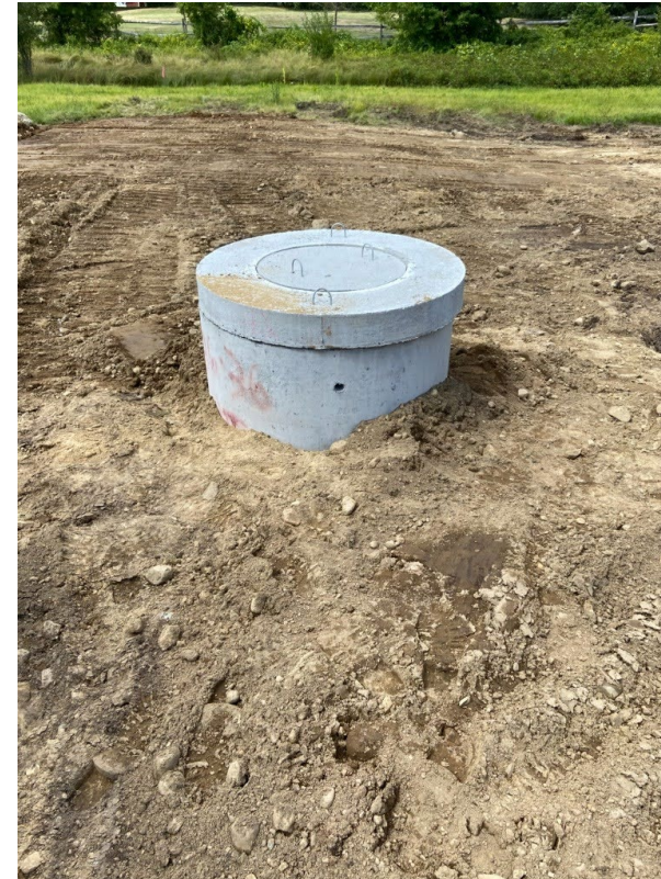
Typical concrete tile dug well
