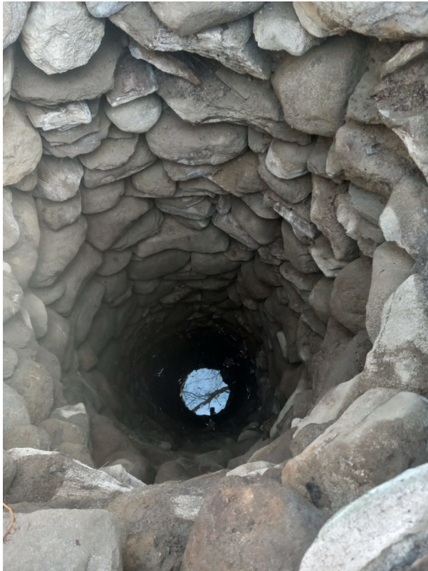
Vintage stone lined hand-dug well
