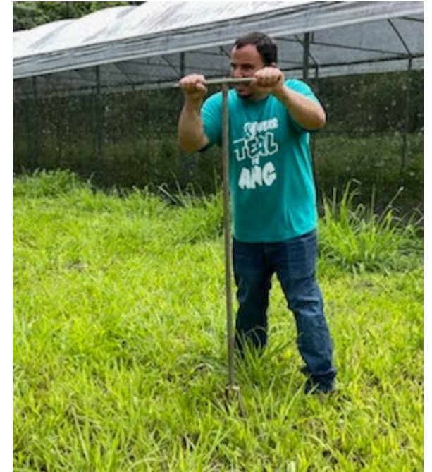
Point wells are often augered by hand and sleeved and pounded in the ground.
