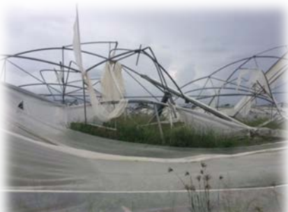
High Tunnel affected by Hurricane Maria
