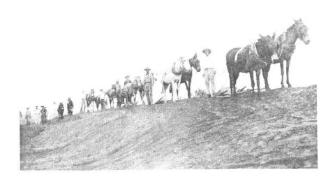
Organized in 1939, the Farm Security Administration, USDA, financed pumps, pipes, and power equipment for the project in 1940. SCS surveyed, designed, and laid out the irrigation system in 1939. Mule teams provided the power to cut ditches and laterals for the distribution system.
